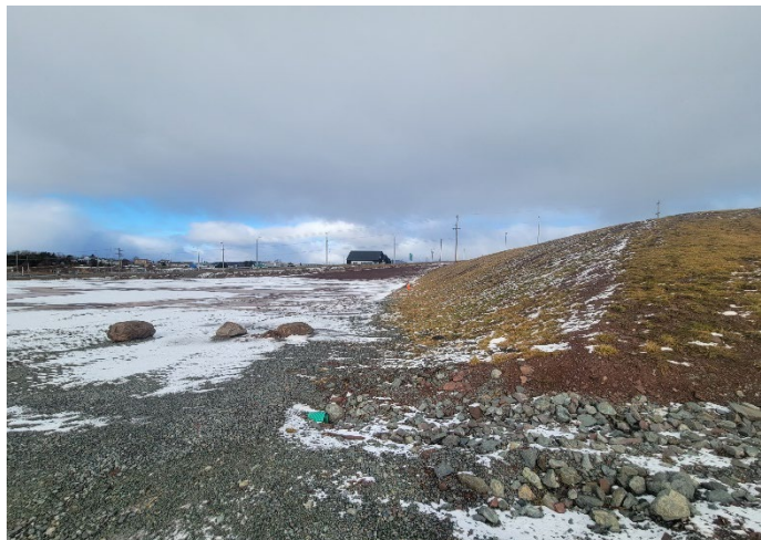
Figure 4. Photo of Site from Site Visit (Jan 11, 2025)
