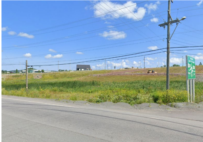
Figure 3. Photo of Site from Google Streetview (July 2024)
