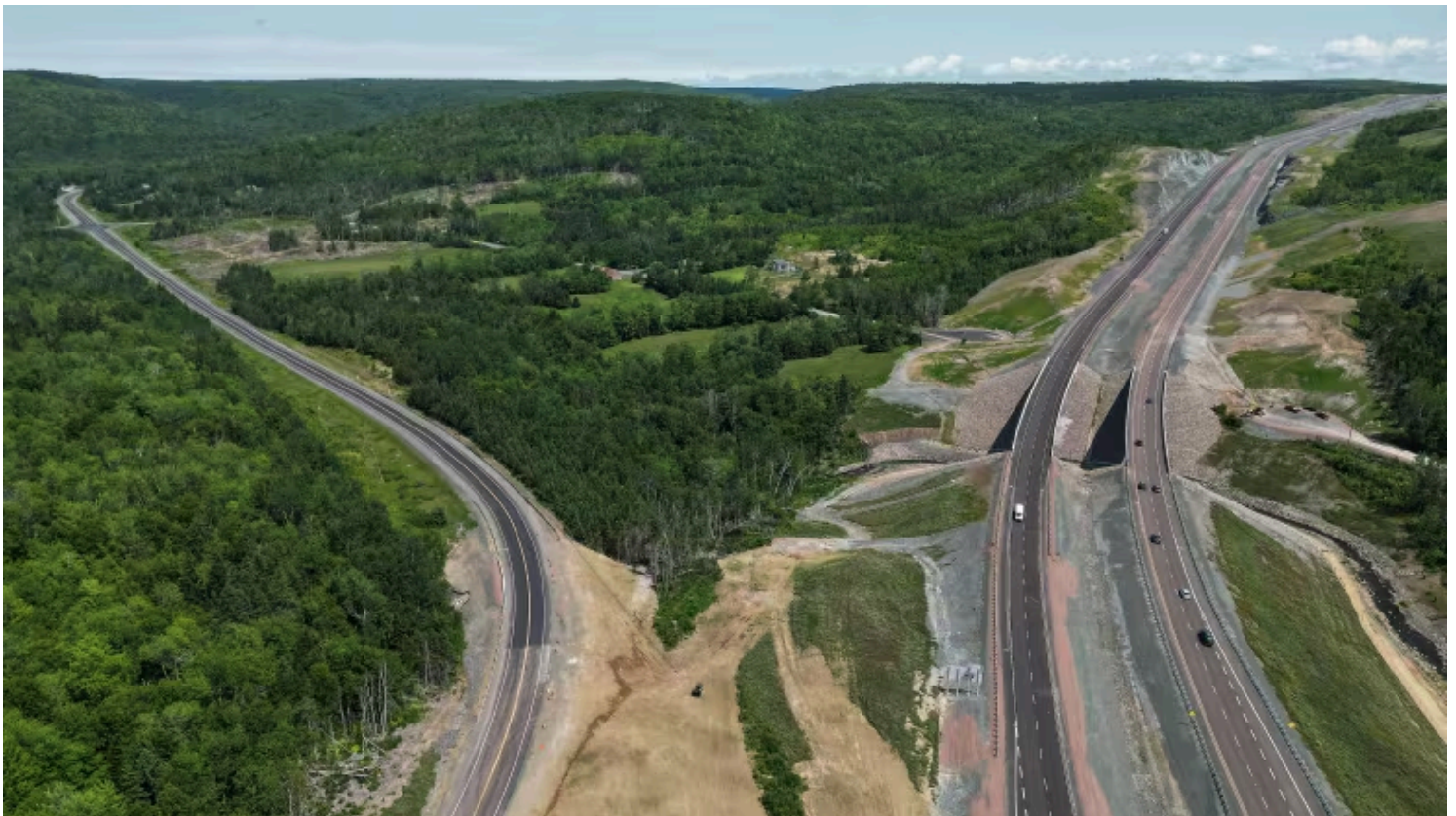
An aerial photo shows the new twinned Highway 104 to the right, and the old single-lane highway to the left. (Communications Nova Scotia)
