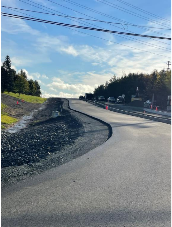
Photo taken from West St. intersection looking East.
