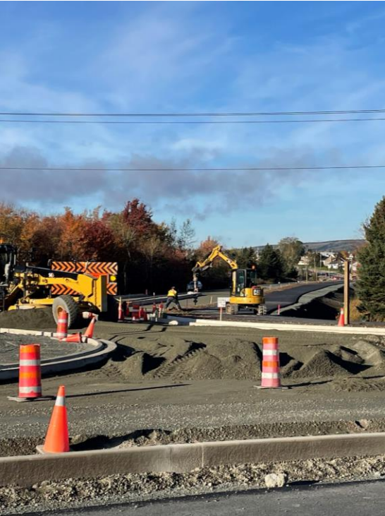
Photo taken from West St. intersection looking West.
