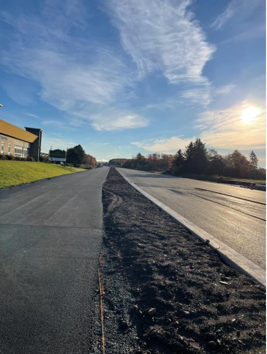
Photo taken from James St. intersection Looking East.
