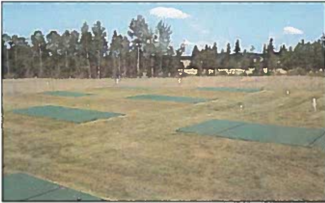
With an Orenco Effluent Sewer, solids are collected in an on-lot underground tank, where they decompose naturally. Only filtered effluent travels to the energy-efficient, low-maintenance treatment system: a modular array of AdvanTex® textile filters in watertight fiberglass containers (above). These textile filters produce such clear, odorless effluent that it is used during the summer for drip irrigation.
